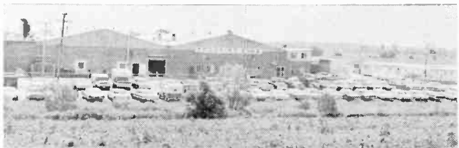
Frontier Industries and Sunset Traveler's plant located on the outer edge of the city.
