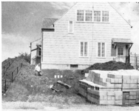
Fall out shelter begun.
