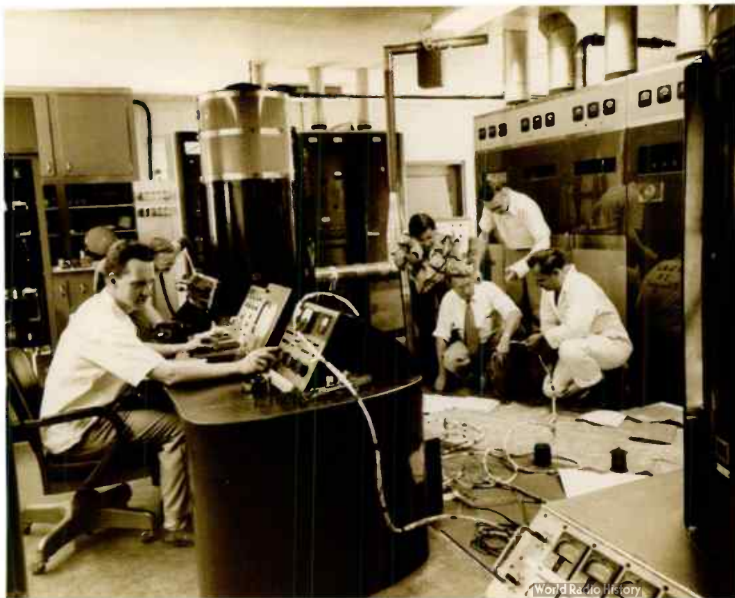
The control room of the new building is being assembled.
