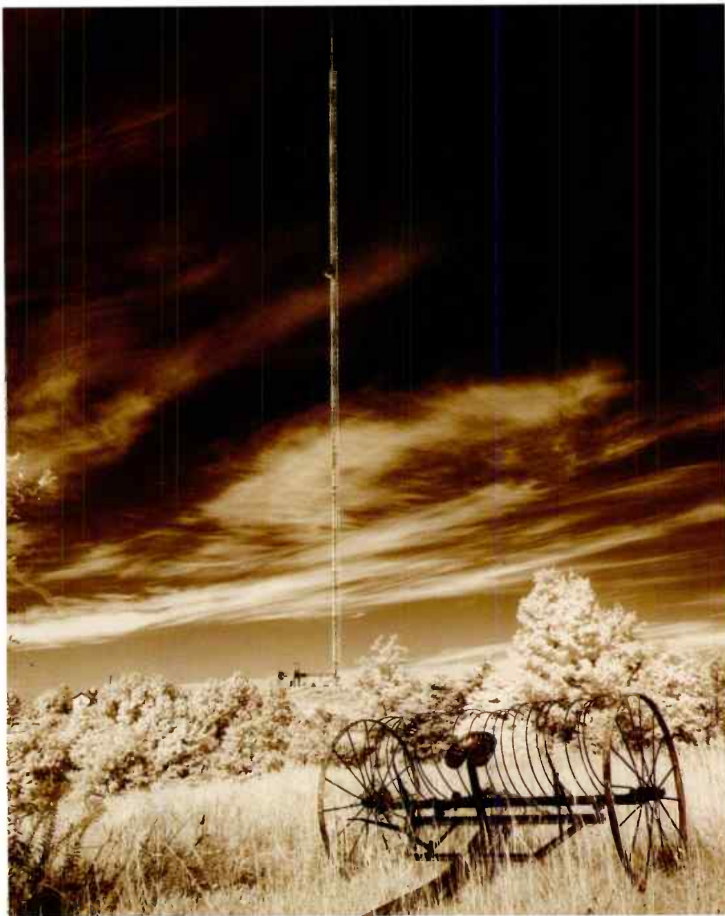
The new 1,000 foot tower.
