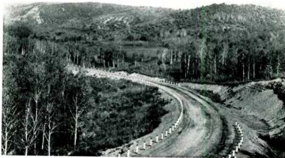
Highway west of Morden.
