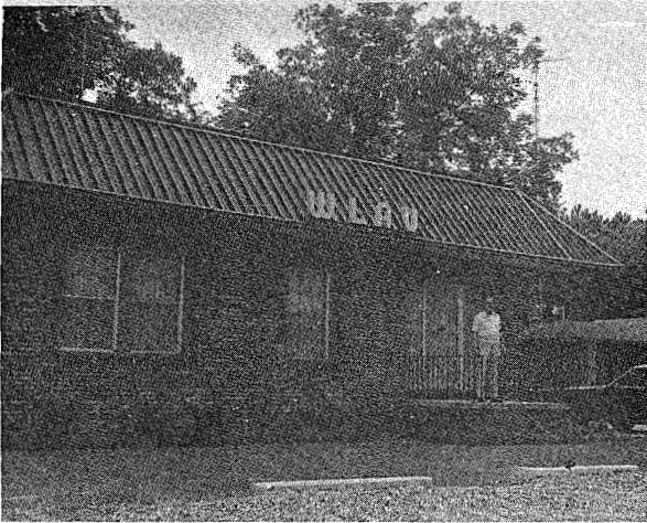
F. M. Smith, General Manager, stands in front of Studio-transmitter-office building of Radio Station WLAU-Laurel, Miss.
