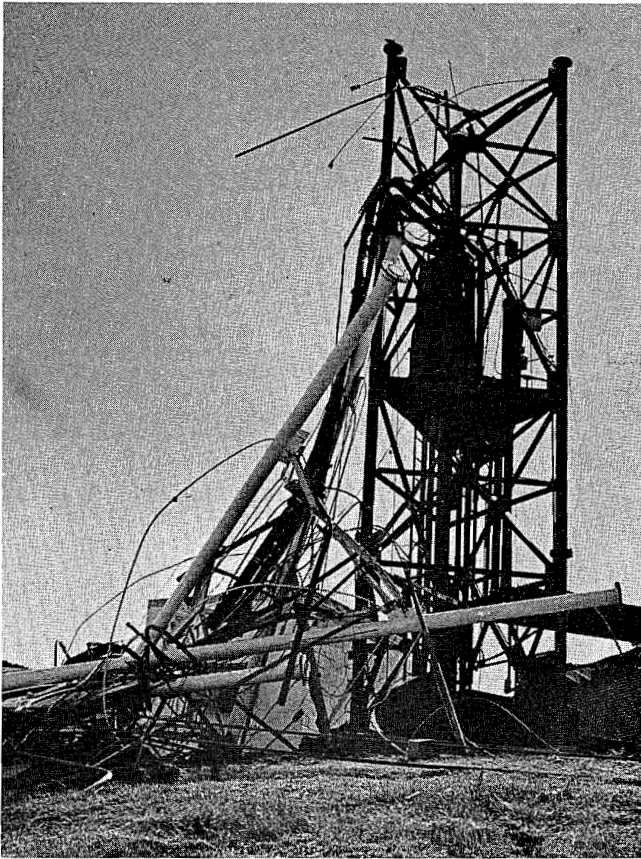
All that remained of the base section of the WLBT-WJDX-FM, Jackson, Miss. 1529 foot tower after the tornado hit. Note elevator in center of tower. [March 3, 1966]
