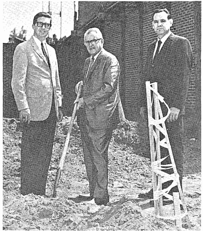
Bob McRaney, Jr. [L], Gen. Mgr. WLBT, WJDX-AM-FM, Floyd Kinard-Chief Engineer, WLBT WJDX-WJDX-FM, turn the first spade in the re-construction of WLBT-WJDX-FM tower destroyed by a tornado on March 3, 1966. At 2,025 feet, the WLBT-WJDX-FM Tower is the tallest tower in Mississippi.
