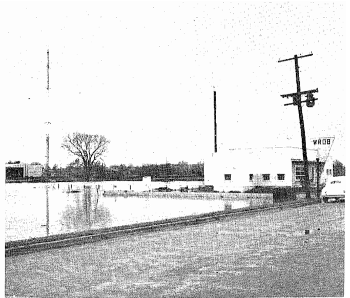
WROB Building-West Point, surrounded by water during local flood-March 19, 1970.
