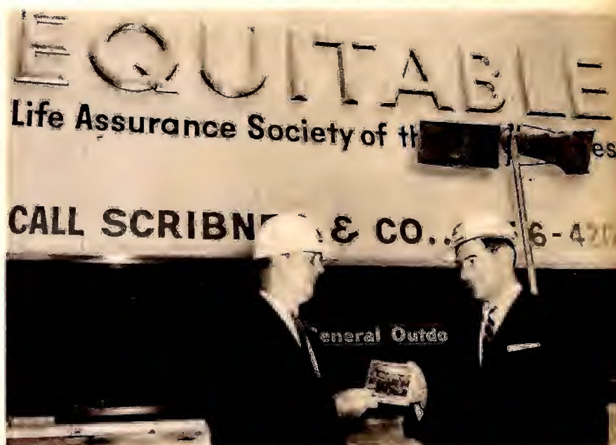
Chicagoans passing the construction site of the Equitable Life Assurance Society on North Michigan Ave. may recognize a familiar voice. Jack Brickhouse (l), mgr. of sports for WGN, made a recording describing the work to be played over loudspeakers, which he presents to William F. Mueller, manager of the impressive project planned by Equitable
