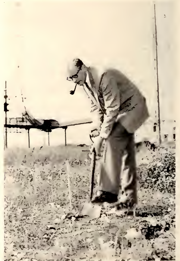
First shovelful for site of new 805-foot WDSM-TV tower (Duluth, Superior) is turned by general manager C. D. Tully. He reports tower will be one of highest structures in Tri-State area
