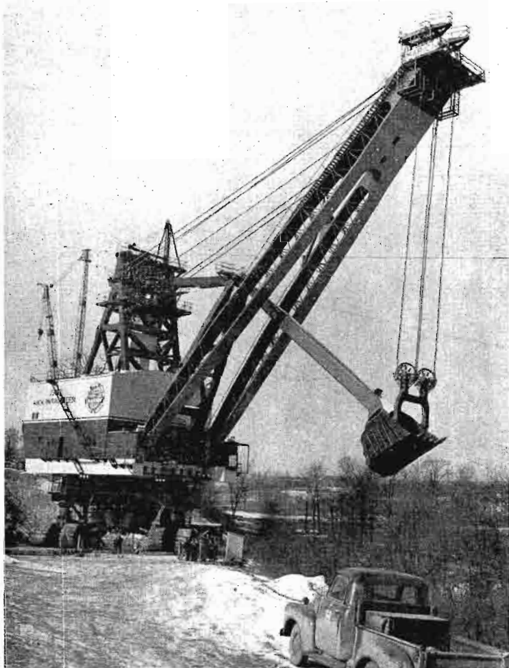
In the Wheeling area lies the nation's only natural supply of coal sufficient for power production necessary for aluminum plants in the eastern United States. Here is the world's largest stripping shovel operated by the Hanna Coal Co. New coal processes now make Ohio Valley power available at prices competitive with Hydrnalic power. Projected underground mines fan out for 30 miles from the Wheeling area.
