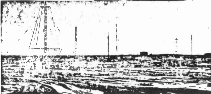
Communications antennas rise sharply above the flat, featureless terrain of the polar plateau.
