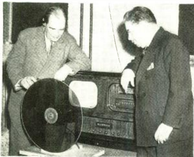
Dr. E. F. W. Alexanderson and George H. Payne, F.C.C. member, inspect the new two-color filter which converts black and white receiver to reproduce colored television images.
