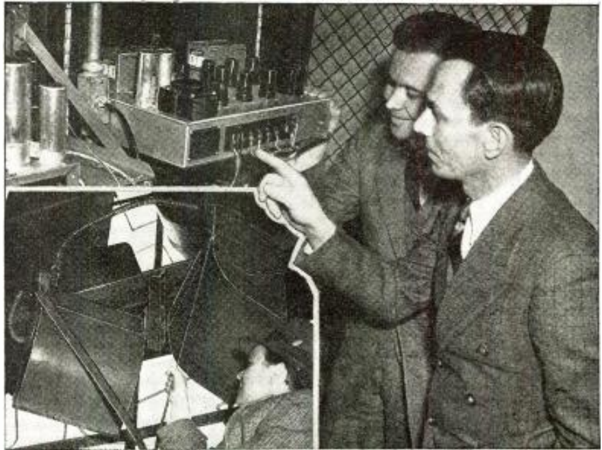
Engineers inspect new chime, Inset—the loud-speaker installation.
