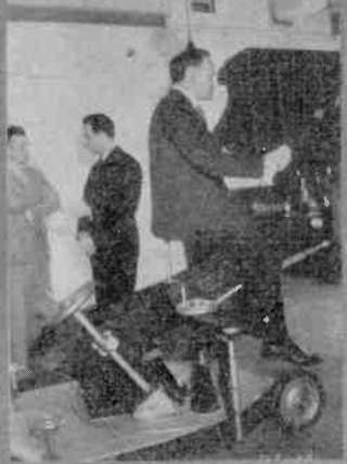
Above—One of the CBS television experts is here seen trying out one of the image pick-up cameras, which is provided with a crane and seat so that the operator can swing around while televising the players in the studio. Frequently two cameras are used, one for close-ups and one for long shots.
