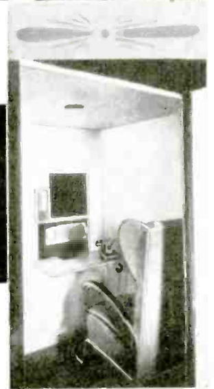
The latest television phone line recently opened between Berlin and Leipzig, Germany, a distance of about 125 miles. The photos directly above show the excellent television reproduction obtained over this 125 mile circuit. The telephone subscriber sits in front of a special image pick-up equipment. (Berlin booth at left), the subject being illuminated by invisible infra-red rays. The photo-electric cell used to pick up the reflected rays is sensitive to these infra red rays. The fluctuating currents corresponding to the variations in the rays reflected onto the photo-cell, are caused to actuate a cathode-ray tube at the receiver.
