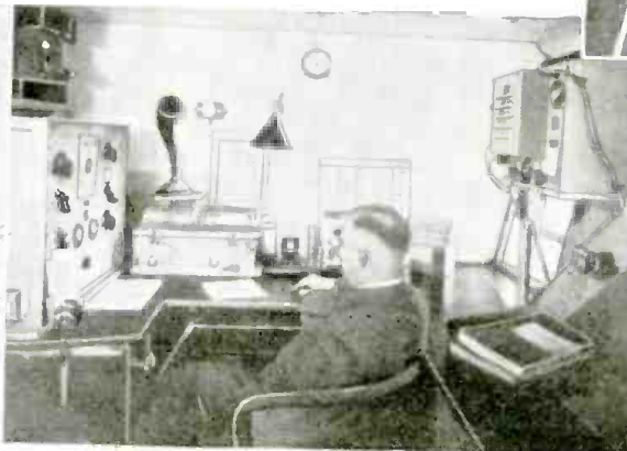
Three photos, left and below—new radio installation aboard German Zeppelin LZ 129. The radio equipment comprises a 200 watt long-wave transmitter, range 600 to 2,000 meters; one short-wave transmitter having a maximum out-put of 150 watts. The wave length range is continuously variable between 15 and 75 meters, and the set is suitable for code or phone. The same type tubes are used in both the short and long wave transmitters, thus simplifying replacement. Two all-wave receivers are provided, having variable range between 15 and 20,000 meters.
