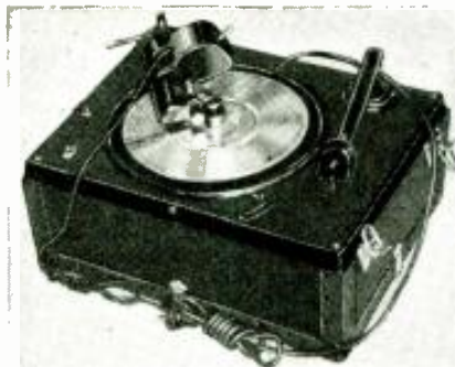
Complete Short-Wave Program Recorder, with Recording Cutter Head and Magnetic Pick-up for "playing back."
