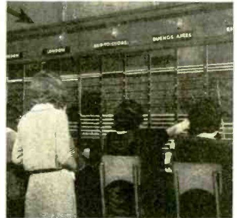
At this switchboard a specially trained group of operators handles all calls between points in North America and Europe, South America and the Far East, as well as to Bermuda and to “ships-at-sea.”
