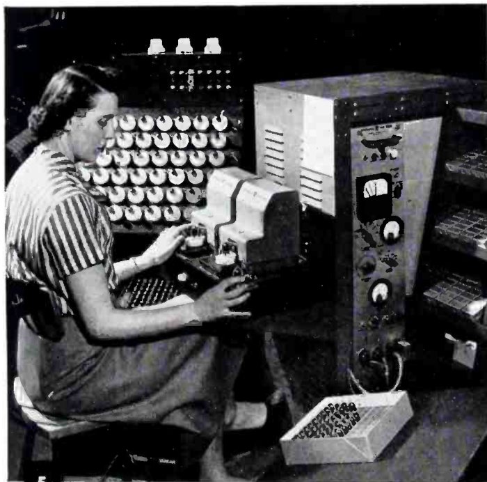
5 —Testing the tester. As a constant check on the accuracy of the automatic tester—samples from each lot tested, are retested on similar equipment used as a standard. Records are kept of all tests serving as data to feed back to design, manufacturing, and quality-control groups.
