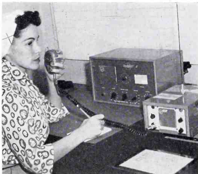
OPERATING one of the fixed two-way installations recently completed by Marine Radio Service.
