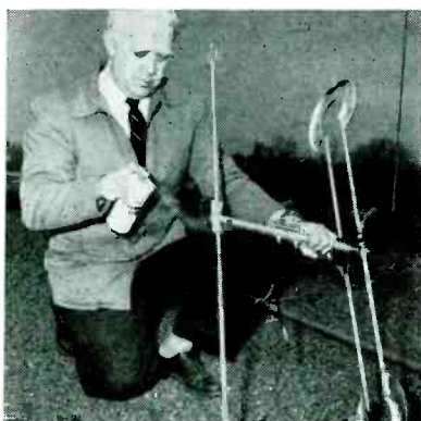
Left: Applying plastic spray to reflector-crossarm point. Center: Another plastic spray application; to standoff insulator and to lead-in section between the antenna insulator and the first standoff insulator. Spray protects standoff and also adds rigidity to the section of twin lead right below the antenna. This minimizes flexing during high winds. Right: Applying protective spray to the antenna crossarm mast-section to prevent rust formation and loosening of the U-bolt section.
