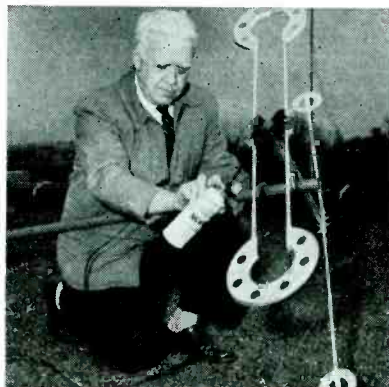
Left: Applying plastic spray to reflector-crossarm point. Center: Another plastic spray application; to standoff insulator and to lead-in section between the antenna insulator and the first standoff insulator. Spray protects standoff and also adds rigidity to the section of twin lead right below the antenna. This minimizes flexing during high winds. Right: Applying protective spray to the antenna crossarm mast-section to prevent rust formation and loosening of the U-bolt section.
