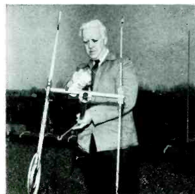
Left: Applying plastic spray to reflector-crossarm point. Center: Another plastic spray application; to standoff insulator and to lead-in section between the antenna insulator and the first standoff insulator. Spray protects standoff and also adds rigidity to the section of twin lead right below the antenna. This minimizes flexing during high winds. Right: Applying protective spray to the antenna crossarm mast-section to prevent rust formation and loosening of the U-bolt section.
