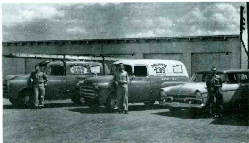
Above: Caldabaugh (right) and his fleet of installation-repair cars. At left is TV-antenna-installation truck. House wagon and second truck are used for service call work.
