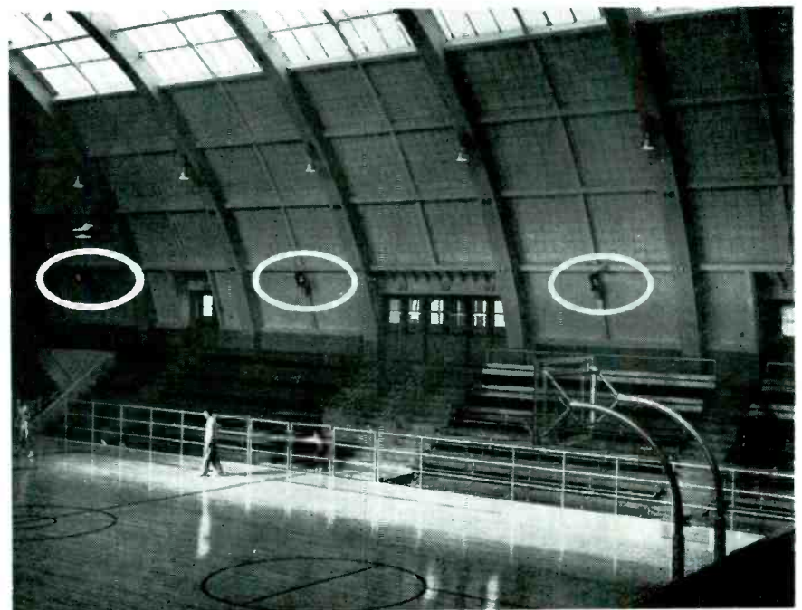
Fig. 4. Beverly Hills High School swim-gym, where half of the playing and seating areas are covered by three speakers near entrances, and three speakers on opposite wall.
