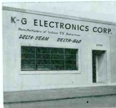
New K-G Electronic Corp. Building
