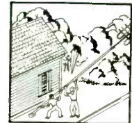
After attaching the antenna, "walk-up" the mast into position and fasten the bracket.
