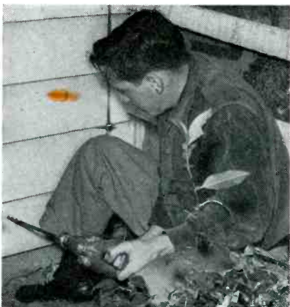
Fig. 4. In drilling hole to basement, drill should be grounded.
