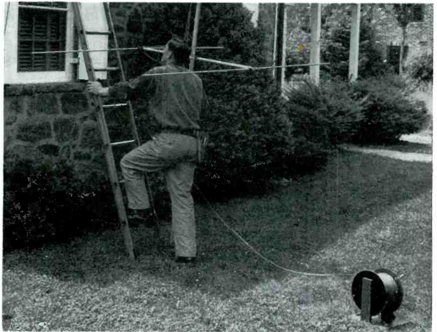
Fig. 3. Use of a transmission line reel-holder which allows the line to unwind freely as antenna assembly is carried to the roof.
