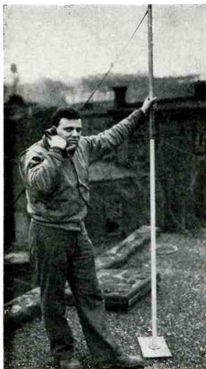
Left: Receiving instructions on orientation of television antenna from Service Man in apartment with test television set. Above: Instructing antenna man how to orient the antenna to secure maximum results on tv receiver.
