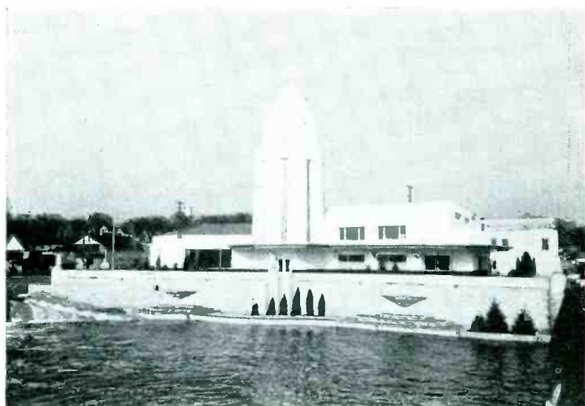
Fig. 2. The main purpose of the amplifying system installed in the Civic Center Building in St. Charles, Illinois, is to supply power for sounding the Westminster Chimes each quarter hour. Provision has also been made for other possible uses, however.
