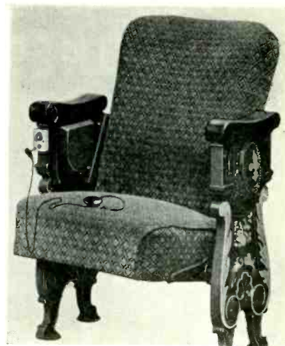
Fig. 1. Showing manner of mounting outlet box on theatre seat.
