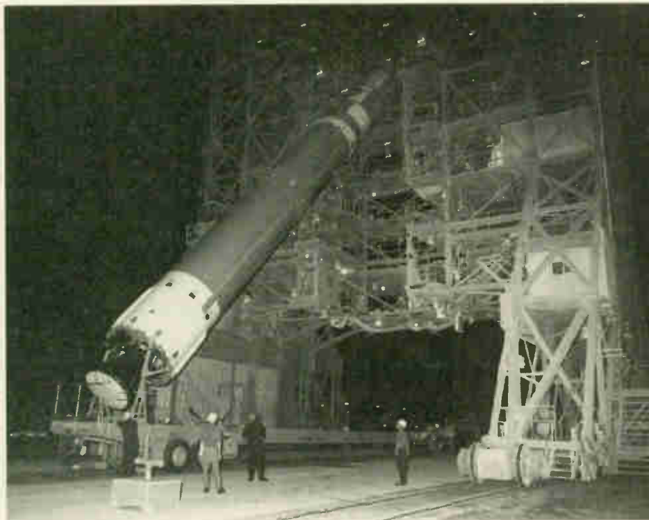
Launch Complex 17, Pad A at Kennedy Space Center. Build-up begins on the Delta II expendable that will carry the Mars Global Surveyor spacecraft. (NASA)
