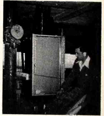
Fig. 2. Outlet box on a vertical conduit with a-c convenience outlet next to it.
