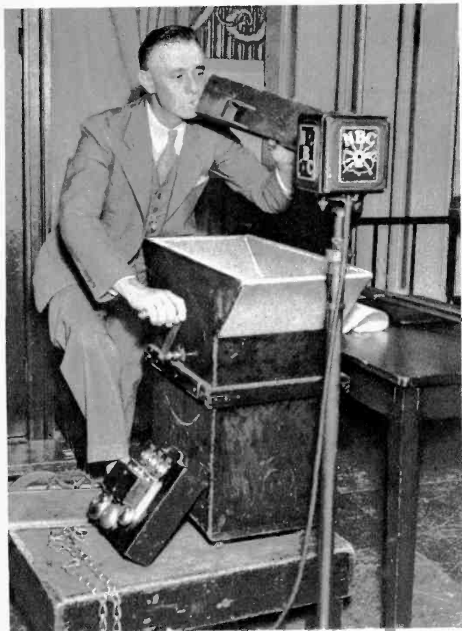
Al Sinton, the sound effect expert, as Old Man Showboat himself. Mr. Sinton is tooting the steamboat whistle and operating the boat paddle which revolves in a small tank of water. Below you see the bell which indicates the rise of the curtain and the chain of the showboat anchor
