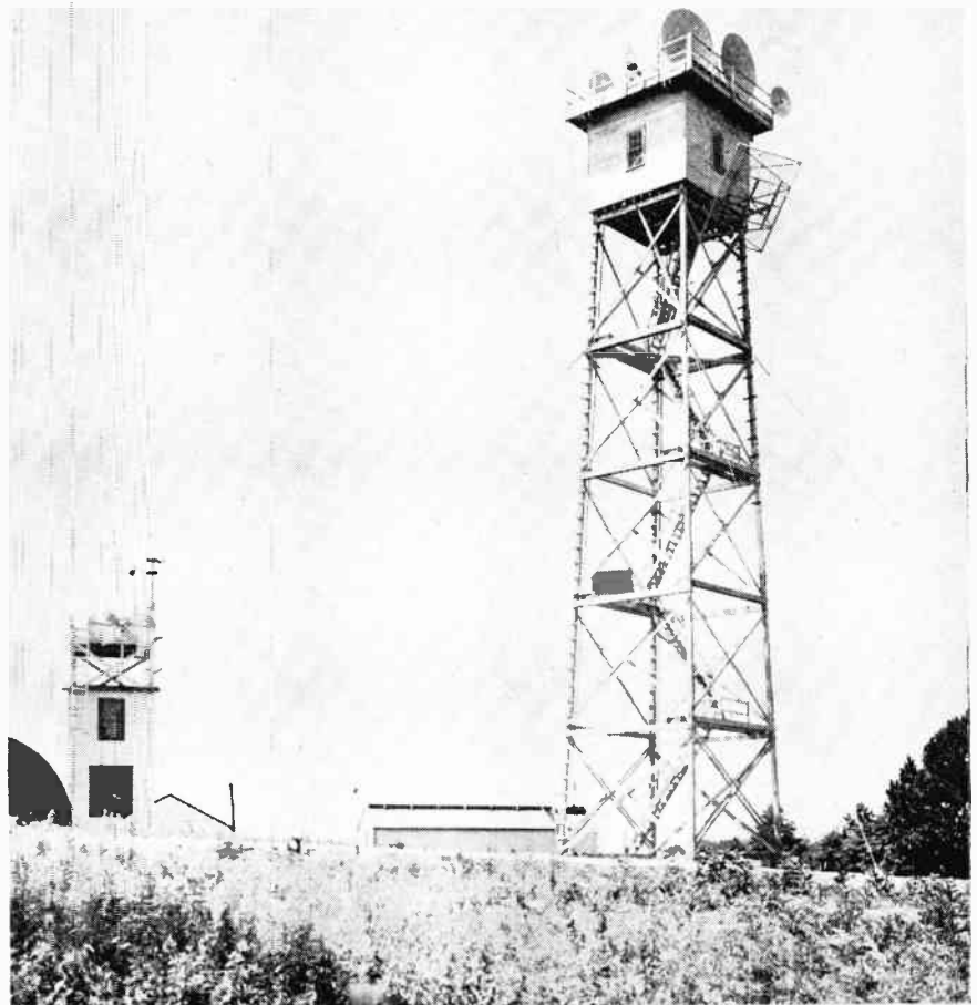
Tower at the Telegraph Hill Field Station with the antenna installation for the PTM Multiplex Radio Relay System developed by the Federal Telephone and Radio Corporation
