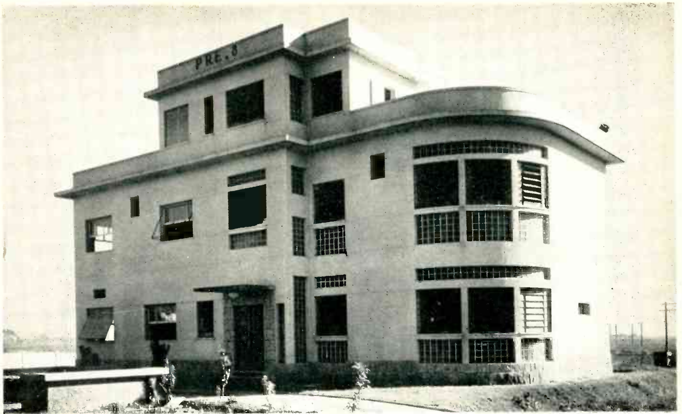
The transmitter building, about 12 kilometers from the center of Rio de Janeiro. The right-hand side of the building is occupied by the shortwave transmitter, and a 25-kilowatt broadcast transmitter is located in the left-hand side.
