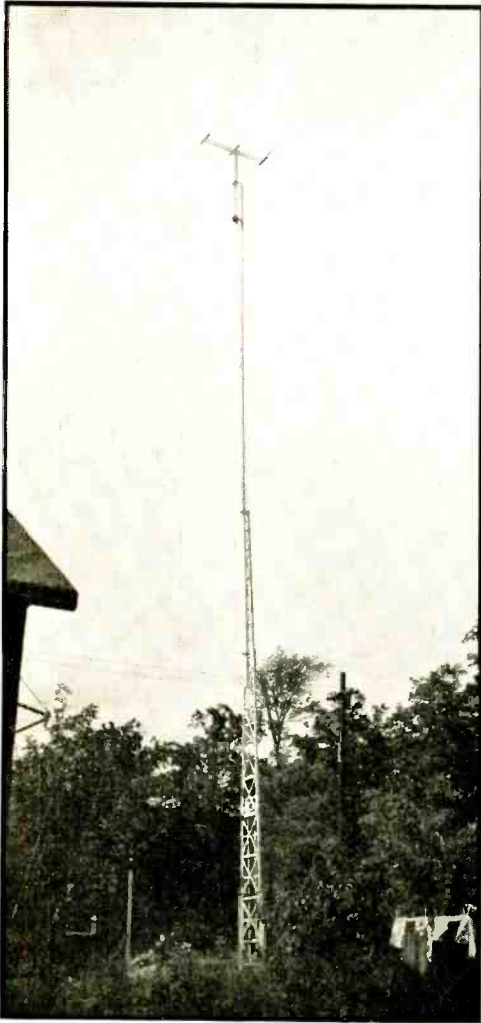
Full length view of the 86-foot light-weight mast in use at W9QCY to support his three-element quarter wave spaced rotary.
