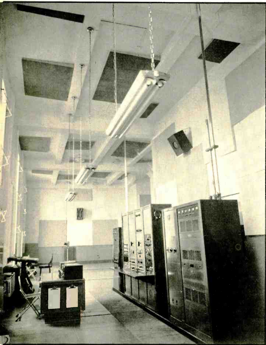
● Overall view of f.m. station W2XOR. Note the "patchwork" acoustic treatment of the room. This is WOR-Mutual's 1-kilowatt f.m. outlet in New York.
