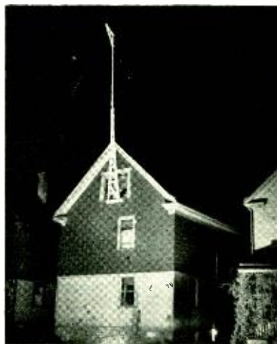
The mast at W8IPD is easily lowered. A block and tackle system into the attic makes it possible to lower the mast and make antenna adjustments with little loss of time.
