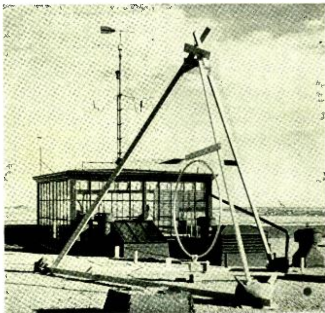
Figure 5. An experimental installation of a static-reducing loop receiving antenna at the Cheyenne ground station.
