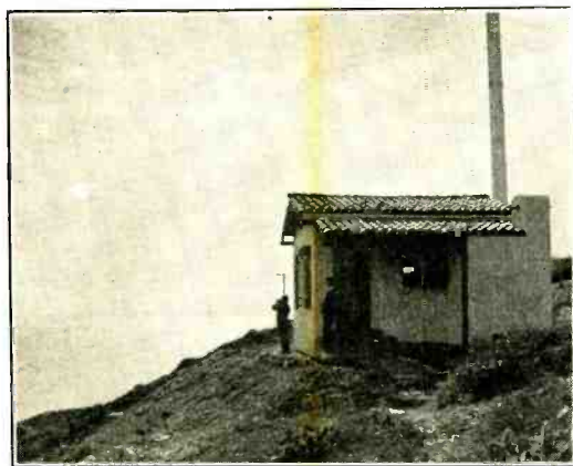
KOU, San Pedro, Calif. Regular telephone service is rendered all manner of boats up to as far as 1000 miles at sea.
