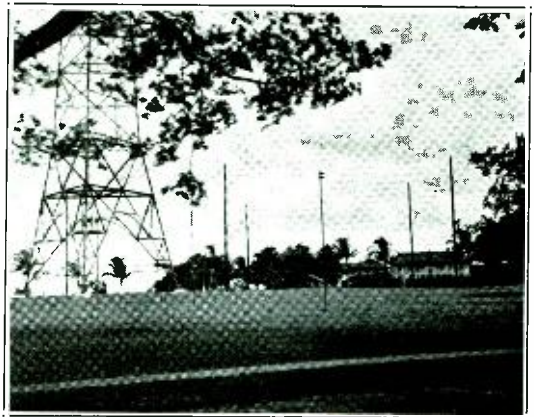
A view of the diamond beams at the Navy radio station (NY1AB) at Balboa, Canal Zone. The short pole in the foreground carries a balanced four wire transmission line which is used with alternate wires connected together. K5AA is located just beyond the buildings, in Fort Amador.
