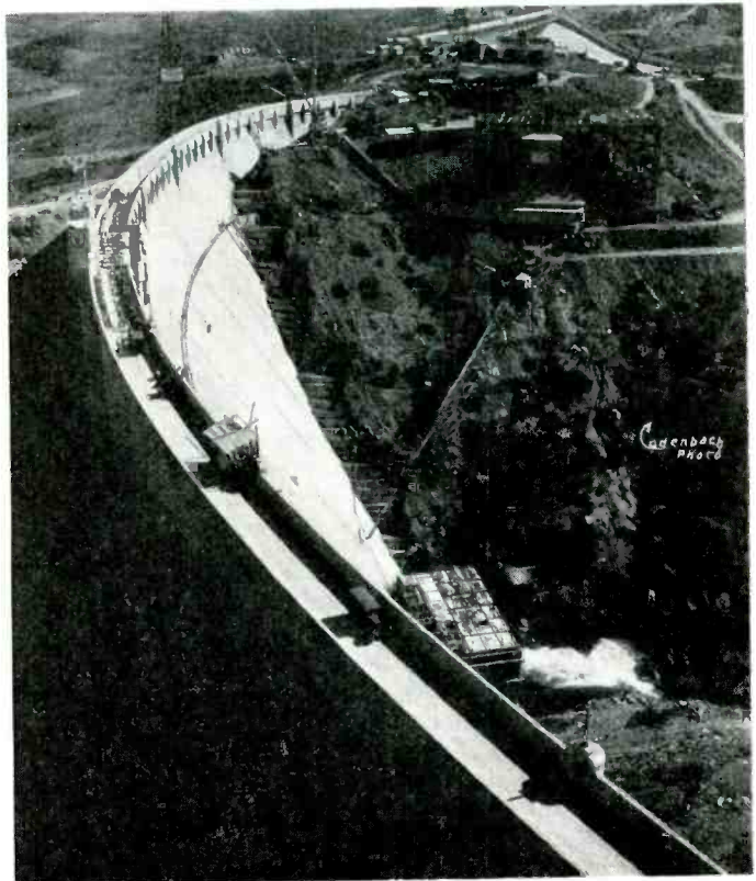
Public Address Installation at Pardee Dam
