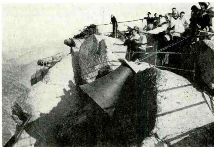
Loudspeaker Installation at Yosemite Valley Fire-fall
