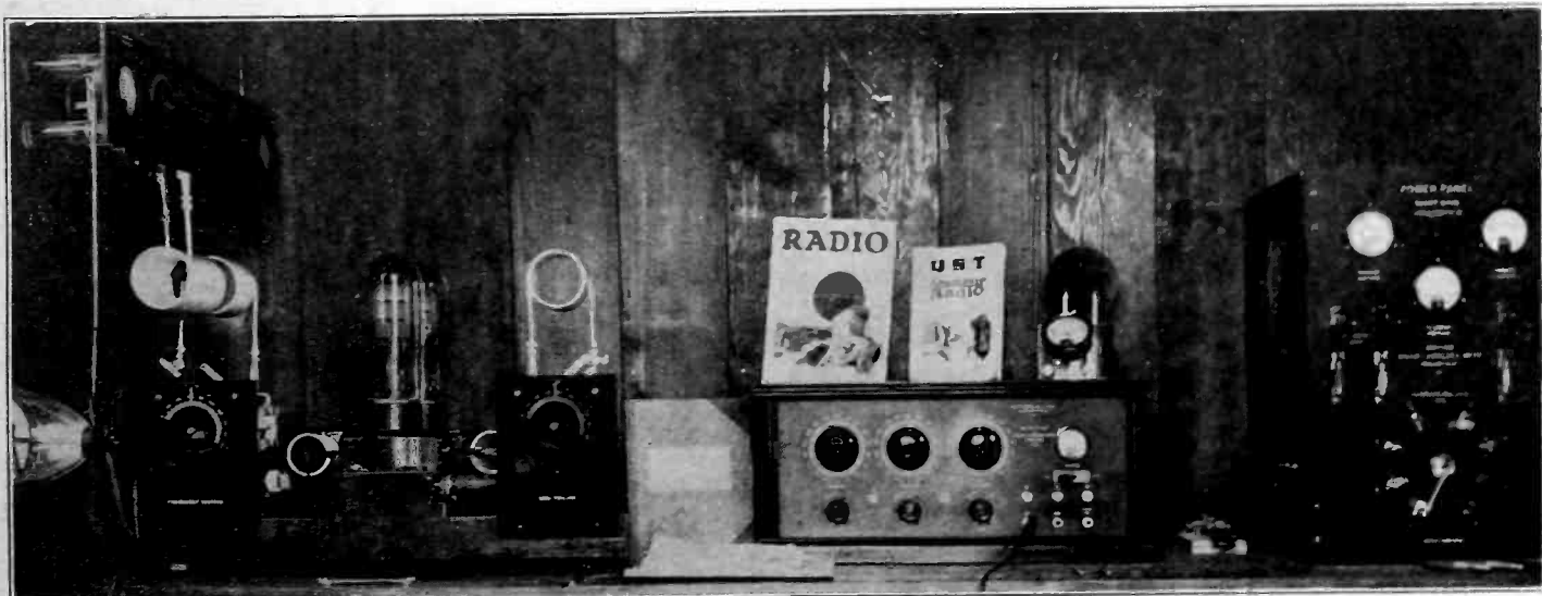
New 500 watt, 5-80 meter Installation at 6XAD-6ZW
