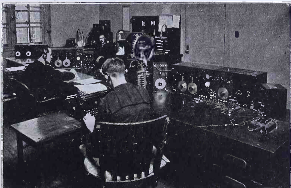
Remote Control Receiving Station at Norfolk, Va.
