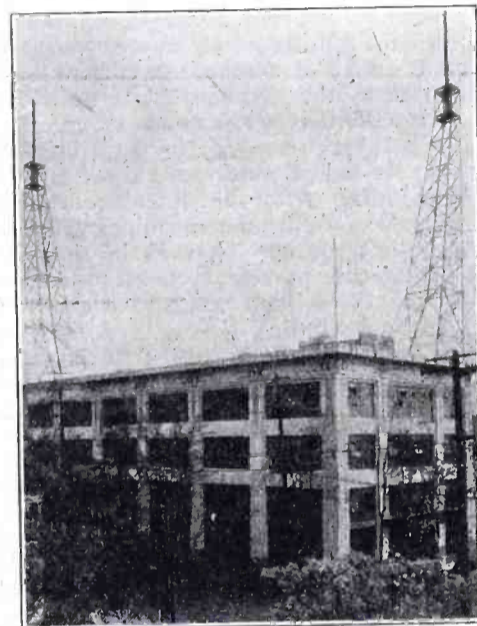
Aerial at KFI Supported by Roof. 96 ft. Steel Towers and 25 ft. Masts so as to be 175 ft. Above Ground.
