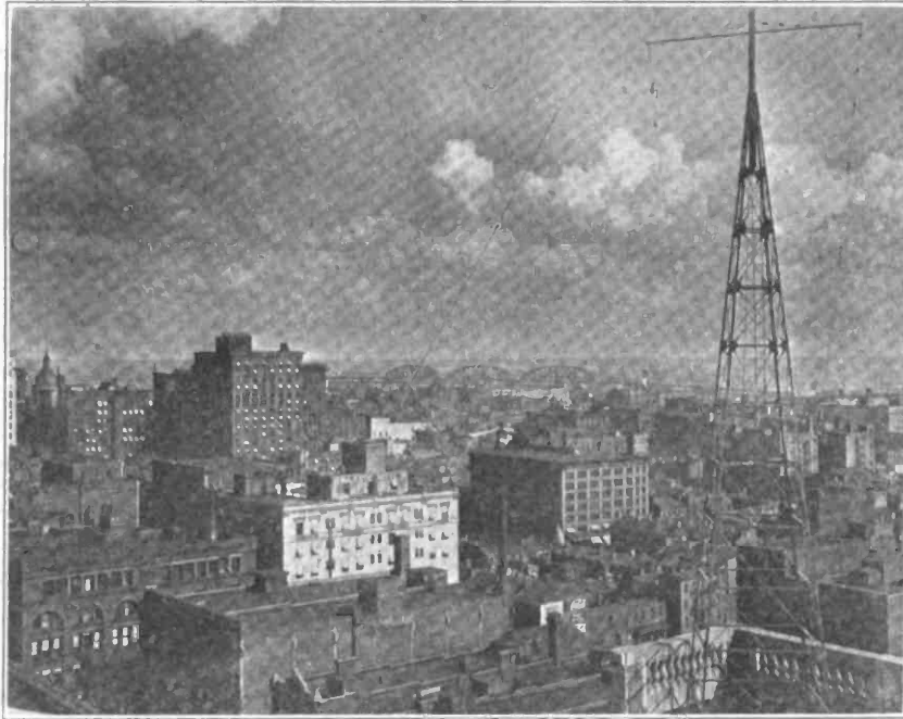
One of the Towers of KSD on the Roof.
