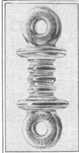
The Brach Crystal Insulator
