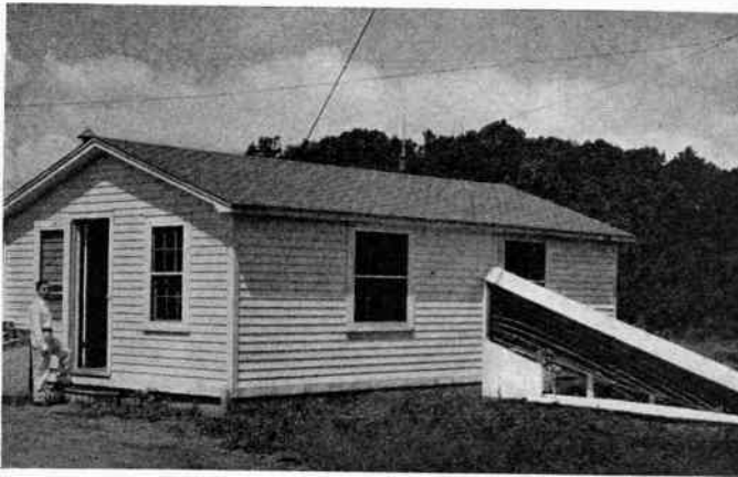
FIG. 1 The musa terminal building and the incoming coaxial transmission lines.
