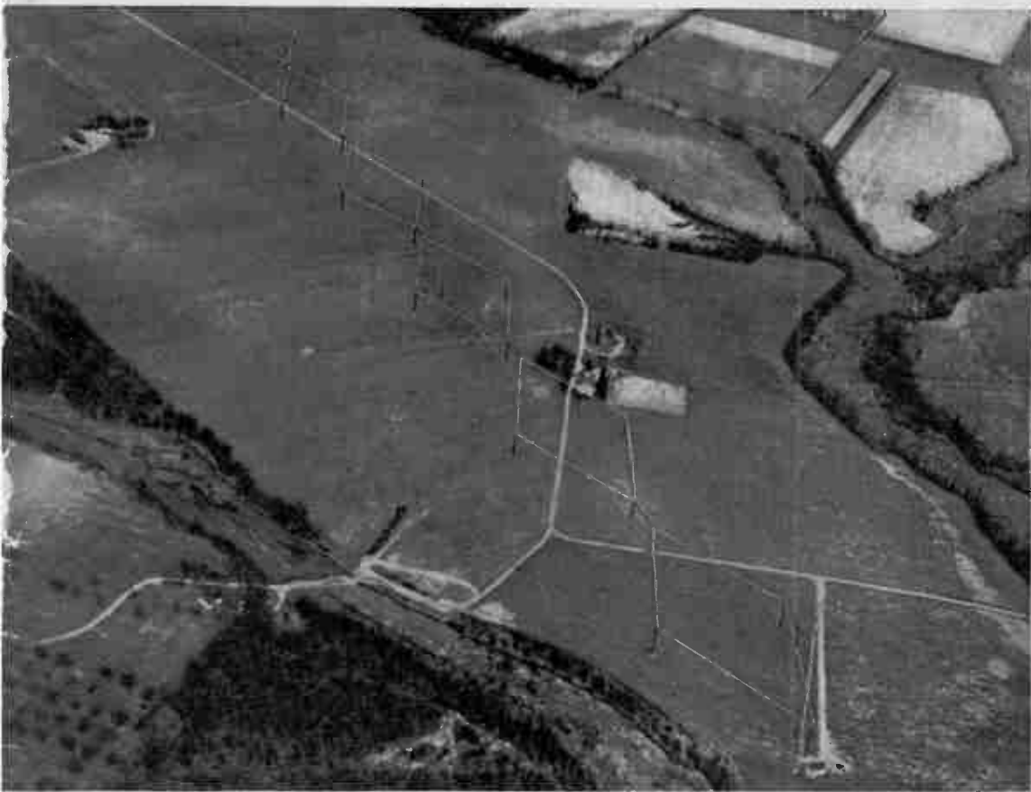
Air view of newly-developed multiple-unit steerable antenna system at Holmdel, N. J., for improving reception on commercial trans-Atlantic circuits. See page 36.
