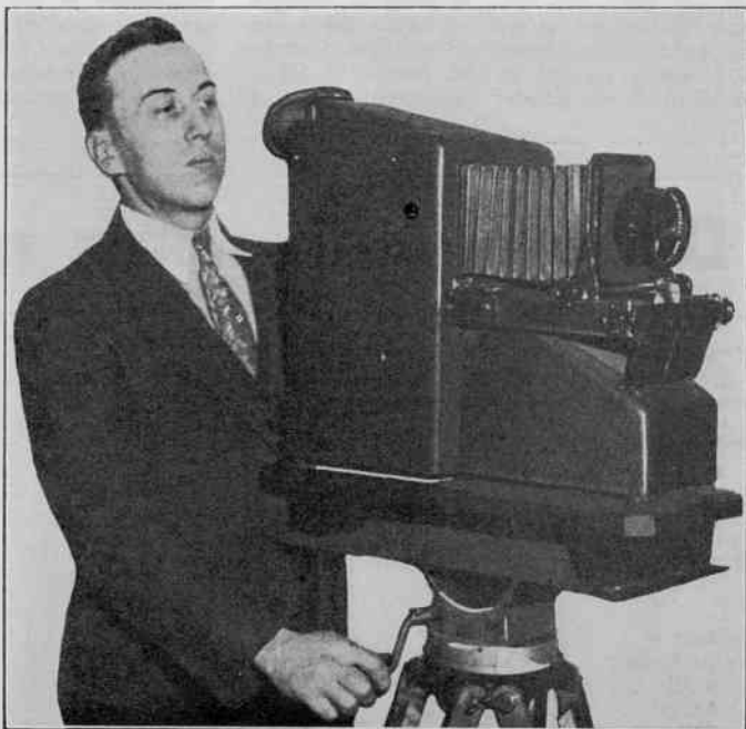
The electric eye of the television camera is being held in the right hand by P. J. Konkle, Philco engineer. Below is the camera, manned by Charles Stee
