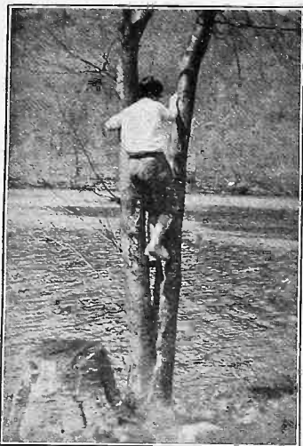
A TREE may be used as an aerial mast, and the usual insulation and other precautions taken for an L-type antenna.
