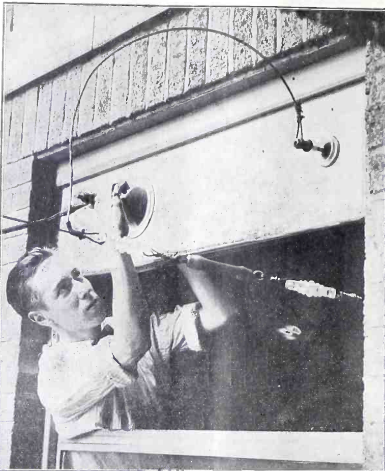
HAROLD HADDEN, of WRNY, "Radio News" station, New York City, adjusting transmitting cable (lead-in) at inverted glass cup, which serves as an insulator. This is the top of an old percolator. (Kadel & Herbert.)
