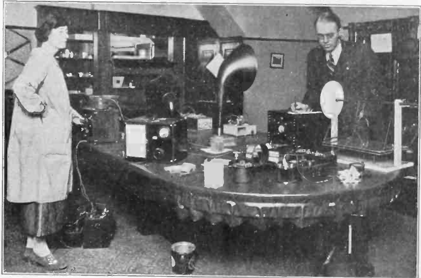
RADIO PARADISE —The laboratory of J. Elliot Jenkins, Chicago radio engineer of international fame. His wife, formerly Miss Alexandra Carlisle, noted actress, is an able assistant to her husband. At the right is a specially constructed condenser with losses that are as near minimum as possible. In plain view, near the condenser, is a wavemeter and oscillator.—(Kadel & Herbert)
