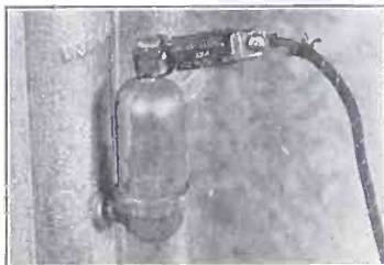
A GROUND spring clamp finds a good gripping surface on the radiator regulator.
