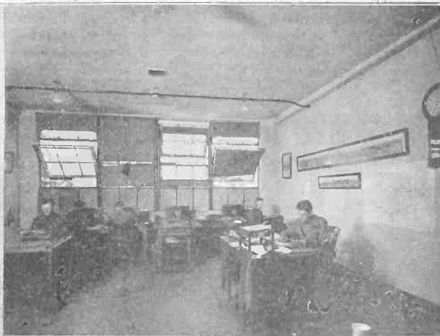
Fig. 2.—Receiving room, Army Message Center, Washington. Messages picked up on the four loop aerials above are brought into the army receiving room to a loop tuner condenser, connected with an amplifier employing three stages of radio amplification, one detector tube, and two stages of audio amplification. Four operators are seen copying incoming messages, and at the right sits Captain R. B. Woolverton, Signal Corps, chief of the Message Center. These men are expert operators and keep in constant touch with all the Army Signal Corps stations day and night.
