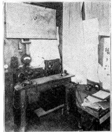
Operating room with receiving set and transmitting remote control
